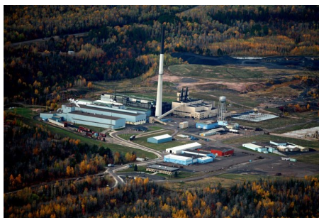
White Pine power plant Source: P.M. Power Group
